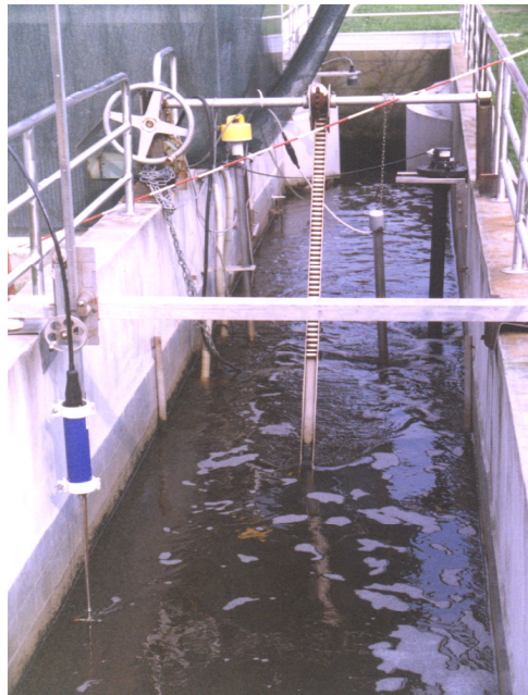
Slika 1: Khafagi Venturi korito na istoku CUP Domžale Figure 1: Khafagi Venturi flume on Domžale WWTP outflow
